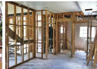
The entire house had to be gutted
